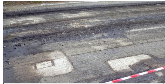
Roadworks revealing anti-tank obstacles on bridge in Shepherdsweil. Photos: Steve Durbridge
